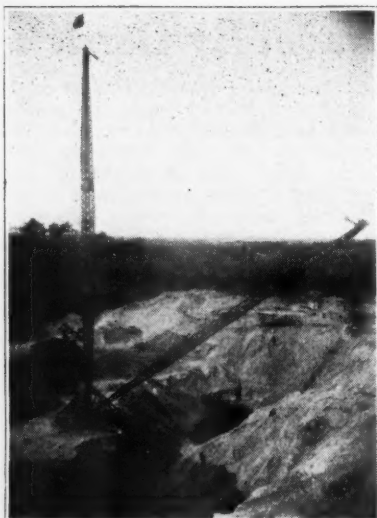
The Derrick Loading Sand and Gravel
